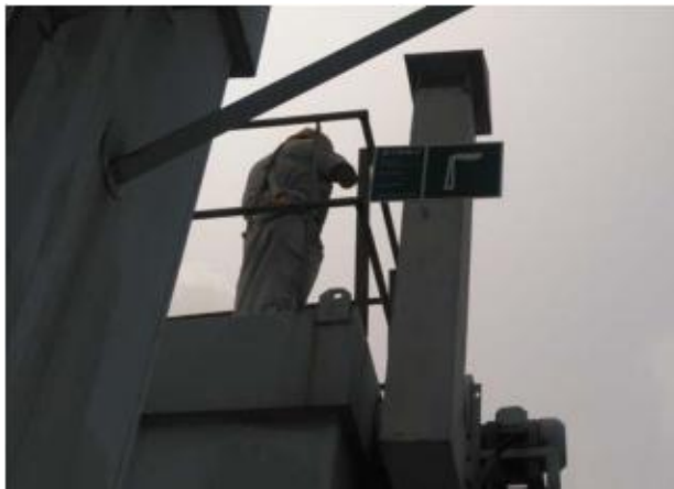
硅灰料仓除尘器排气筒 P 3
